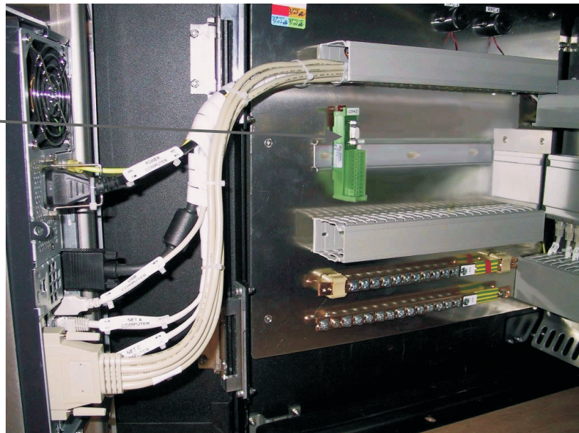
Figure 31 Terminal board – new type
