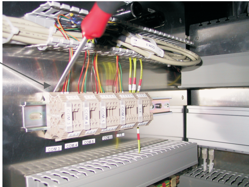
Figure 30 Disconnecting old termination board
