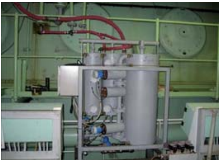
Fig. 55: Measuring tanks for cooler casing drains
