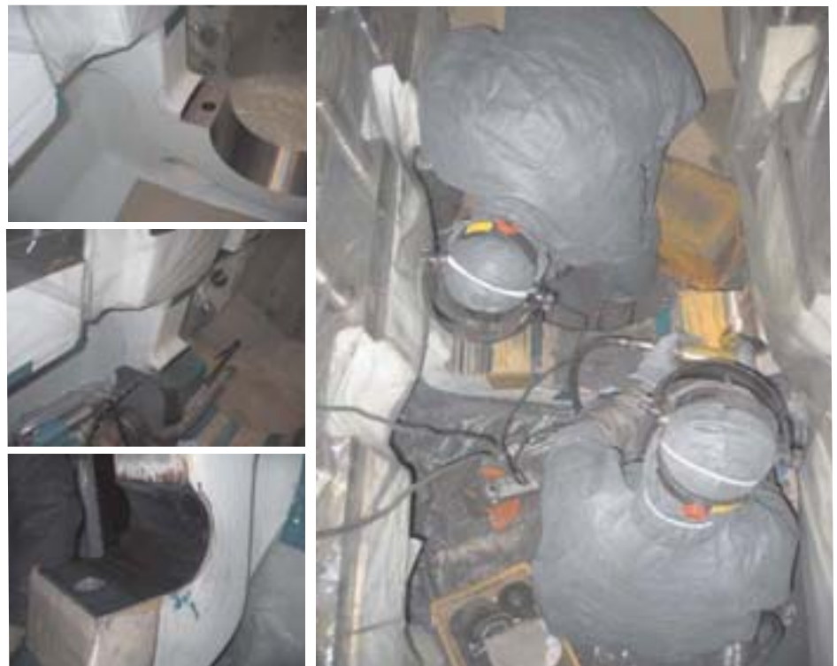
Fig. 69: 'Hand machining' of camshaft housing bearing pedestal roundings
