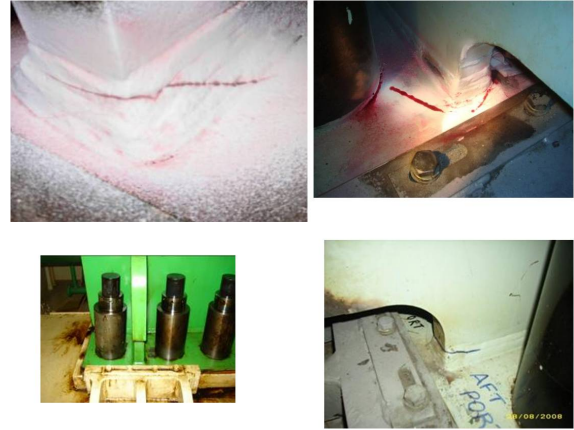
Figure 25 – Lifting bracket cracks
