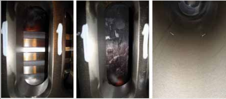
Fig. 24: Scavenge port inspection
