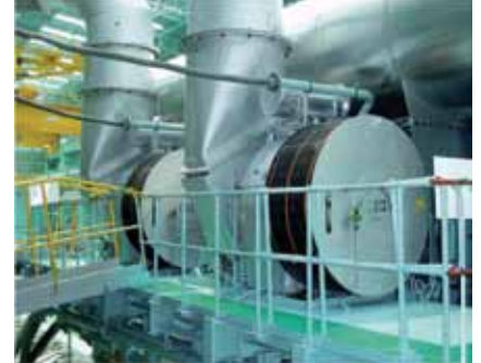
Fig. 51: Modern turbocharger enabling more than 30,000 hours between major overhauls
