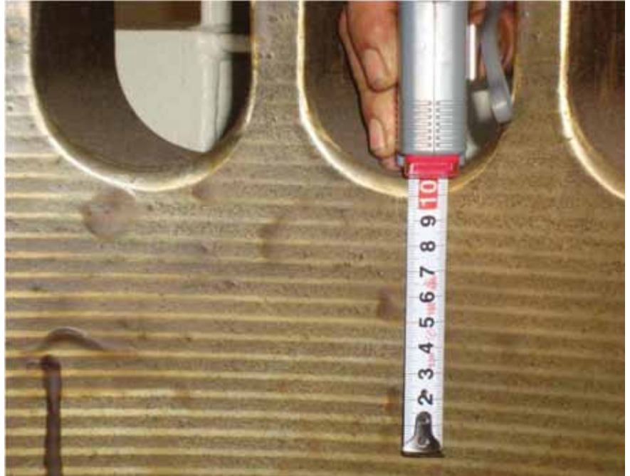
Fig. 31: Cylinder liner quality: insufficient plateau honing
