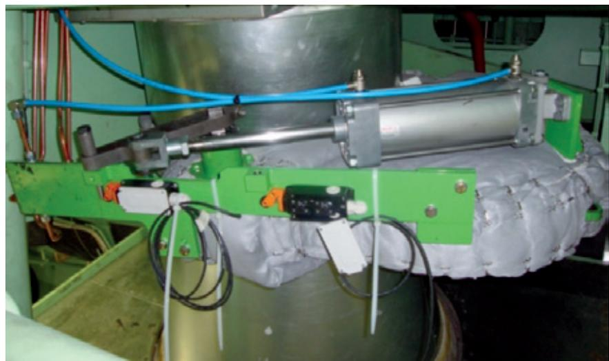
Fig. 18: T/C cut-out valve (compressor side)
