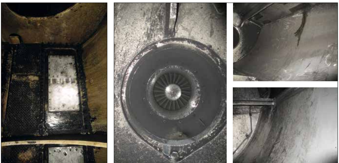
Fig. 42: Blanking of non-return-valves
