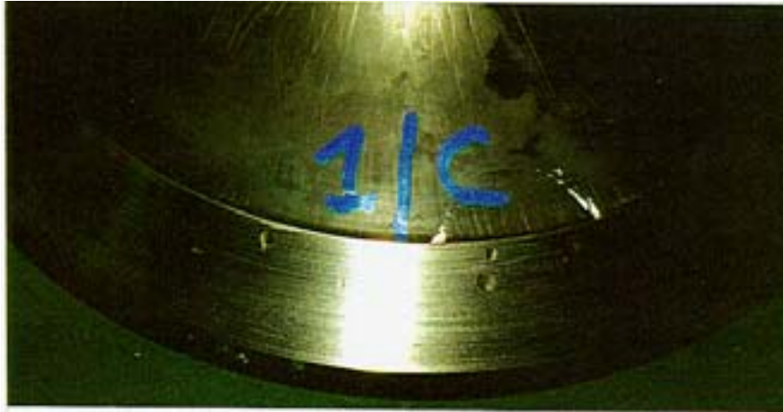
Photo 5: Acceptable seat condition after grinding
