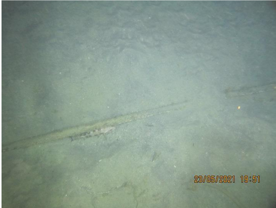
Image 8: Fiber optic cable NC 6
