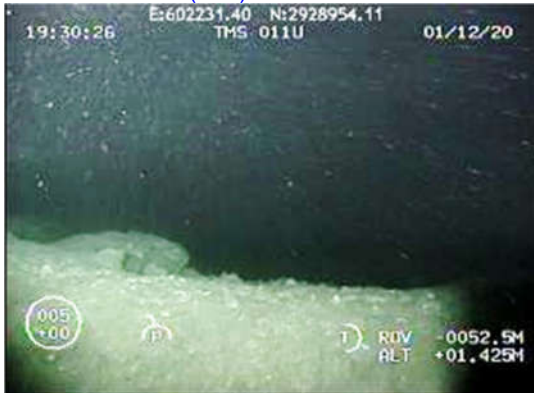
Seabed depression (fix-5)
