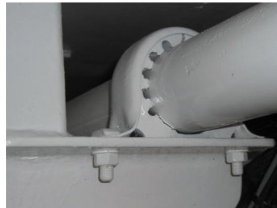
Pipe clamp type delivered from 2007 onwards
