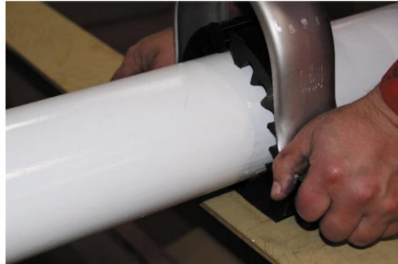
Re-install the pipe clamp steel body.
