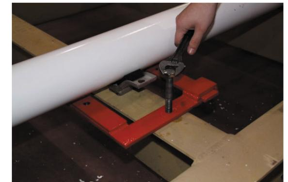
Lift the pipe off the rubber element by turning the bolts.
