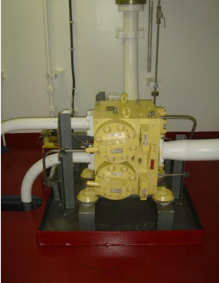
DSTC-80 (Directional Speed/Torque Controller) and solenoids for directional- and speed control
