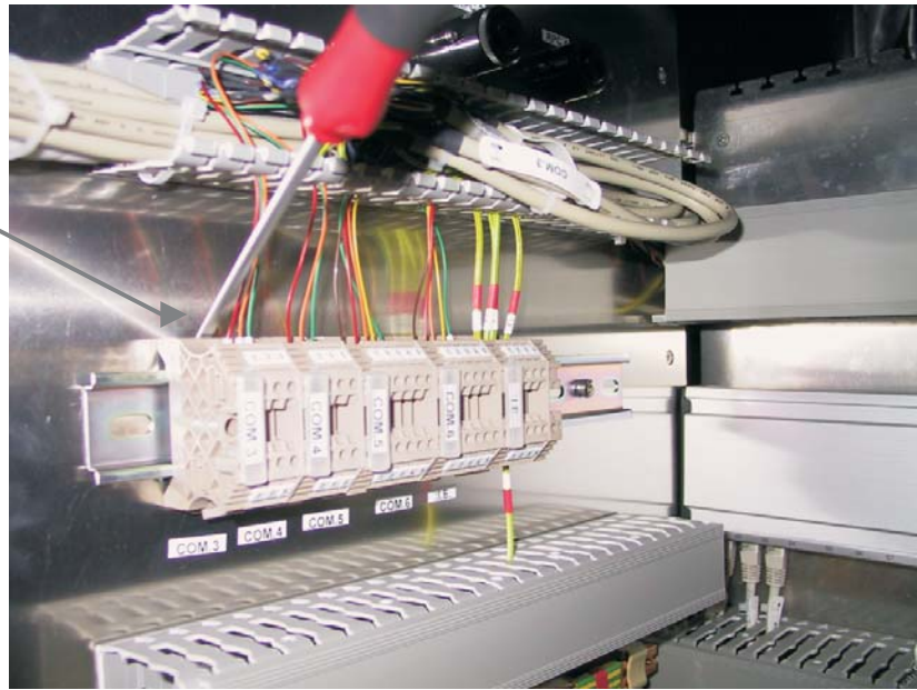
Figure 30 Disconnecting old termination board
