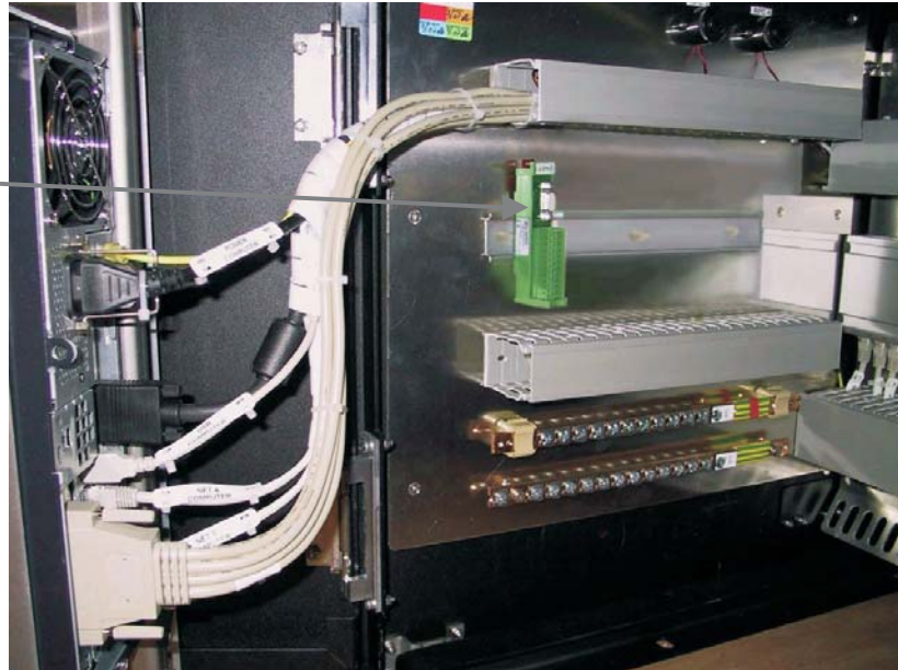
Figure 31 Terminal board – new type
