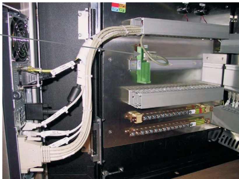
Figure 32 Typical MP7600 w/8 channel system (new terminal board)
